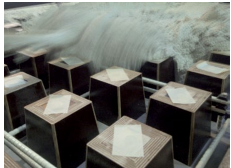
Individual formwork construction
