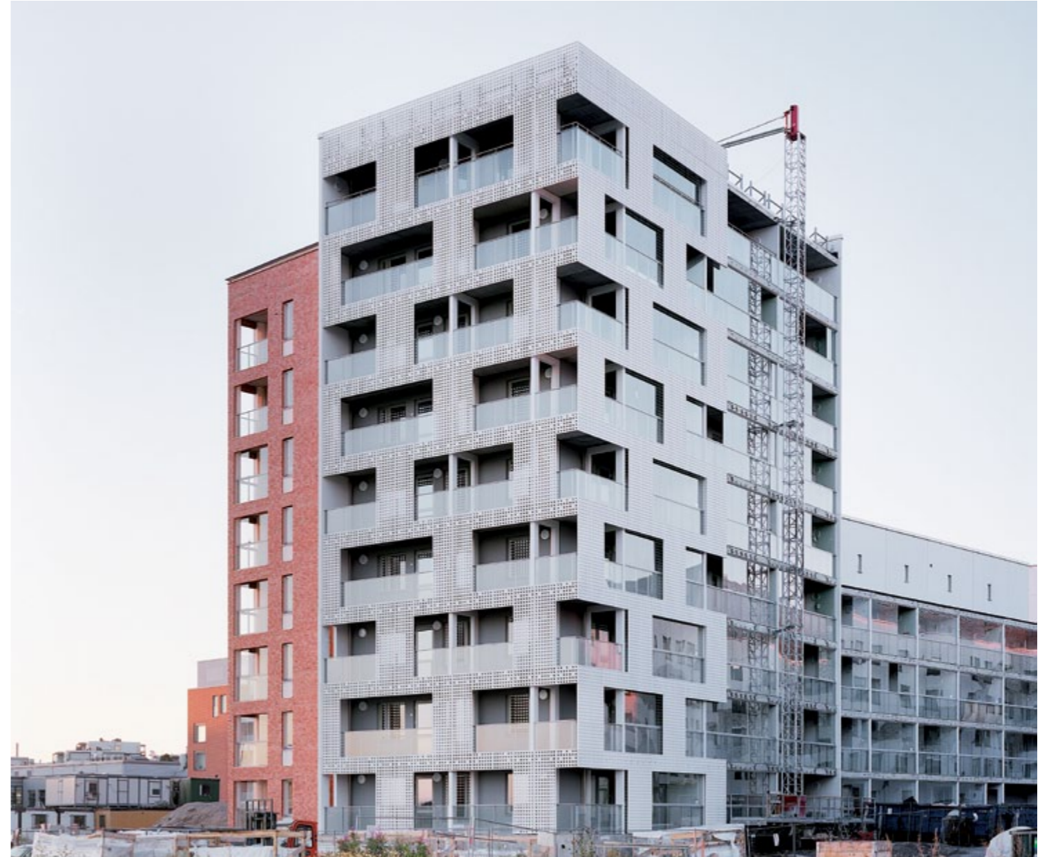
550 m 2 fibreC 3D elements with a thickness of 7 cm are cladding the Lontoonkatu 9 project in Helsinki, designed by Kirsi Korhonen and Mika Penttinen Architects. The entire facade was divided into 16 different types of panels with lengths up to 3.8 m. More than 400 concrete elements with faced concrete quality on both sides offer an interesting view from inside of the building.
