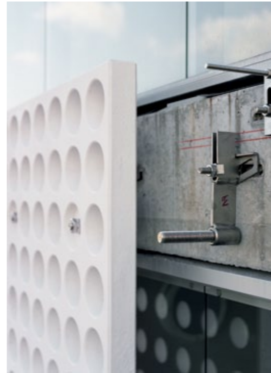
550 m 2 fibreC 3D elements with a thickness of 7 cm are cladding the Lontoonkatu 9 project in Helsinki, designed by Kirsi Korhonen and Mika Penttinen Architects. The entire facade was divided into 16 different types of panels with lengths up to 3.8 m. More than 400 concrete elements with faced concrete quality on both sides offer an interesting view from inside of the building.
